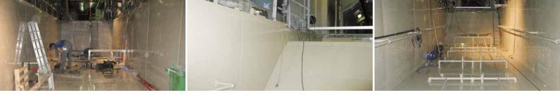
From left to right: applying the SIMONA® PP AlphaPlus® lining to the cathodic electrocoating bath; bath overflow; installing the nozzle pipes
