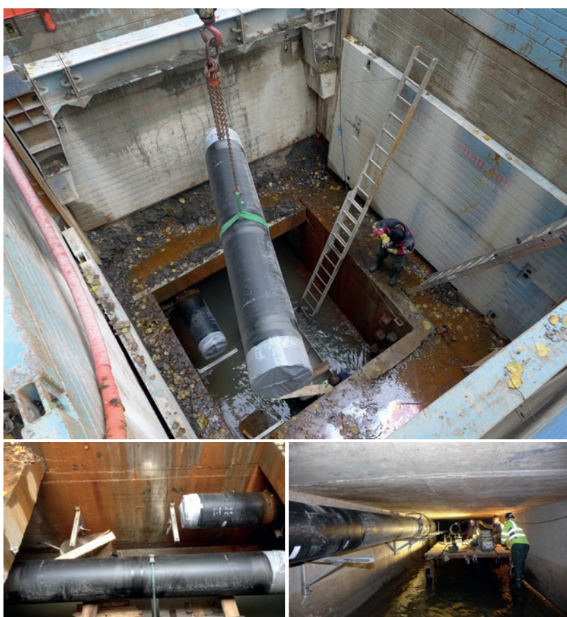
Top: Sinking the SIMOFUSE® pipe modules via the access structure. Bottom left: Transporting the pipe modules on specially built trolleys. Bottom right: Mounting the SIMOFUSE® pressure pipeline in the underground stream section
