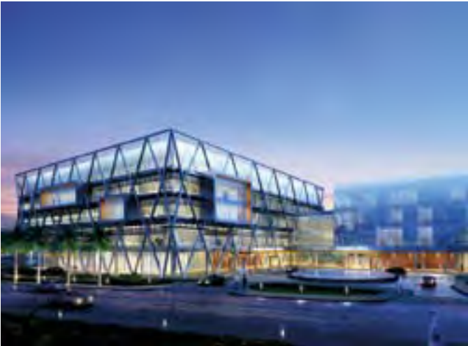
Arzanah Medical Complex - Abu Dhabi (United Arab Emirates)
