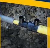
'17.5 mm system, the relining solution for ¾" service pipe'
